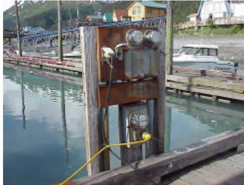
Most of the supply side of the electrical distribution system on shore has been upgraded and/or replaced to accommodate future upgrades. It is in good condition and should require only minor modification when float and electrical distribution systems are replaced or upgraded in the future.
